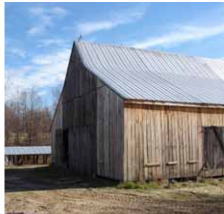
Phipps barn with recent repairs and new siding.
