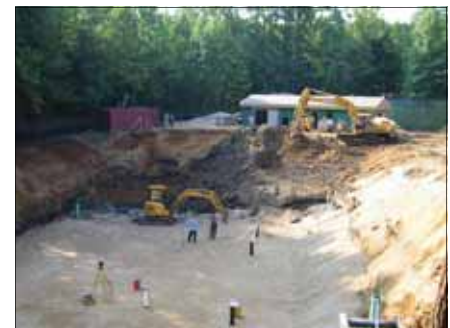
Wastewater Treatment Plant Construction
