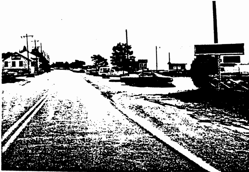
FIGURE 30 - "TIDEBOX" BRIDGE AT THE SOLOMONS ENTRYWAY (1984)
