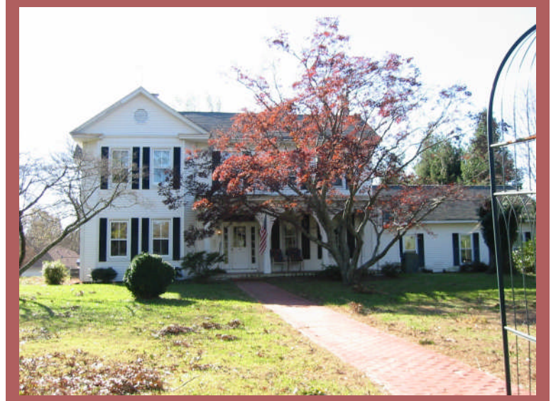
CT-753, on Huntingtown Road, began as a smaller house about 1840, and took on its Victorian appearance around 1900. It belonged to Dr. Leitch
