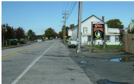
Figure 17: Existing Sidewalk Condition (non-existent)
