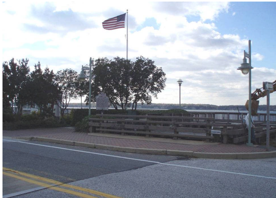
Figure 12. “TIDE BOX” BRIDGE AT THE SOLOMONS ENTRYWAY (2007)
