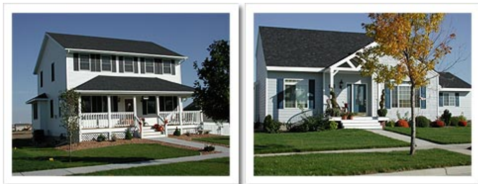
Model Homes at Tallgrass Village, a small mixed-use development in suburban Brandon, SD.
