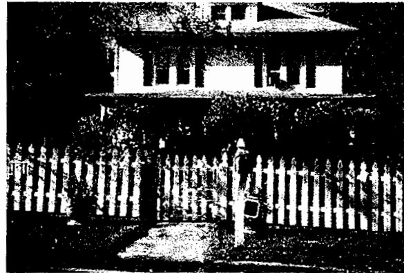
Figure 4-3 This house on Old Solomon's Island Road in Owings utilizes a "Fence and Porch" frontage to enhance the public space of the street while clearly delineating a private front yard, a space from which to greet neighbors on a stroll.
