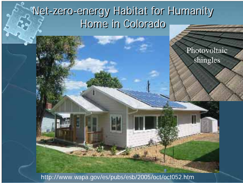
Habitat for Humanity partnered with National Renewable Energy Laboratory to build its first true net-zero-energy home in Wheatridge, Colo. (Photo by Pete Beverly ) http://www.wapa.gov/es/pubs/esb/2005/oct/oct052.htm
