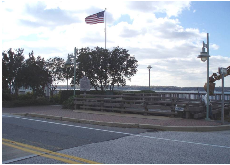
Figure 12. “TIDE BOX” BRIDGE AT THE SOLOMONS ENTRYWAY (2007)
