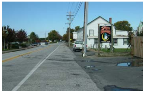
Figure 17: Existing Sidewalk Condition (non-existent)
