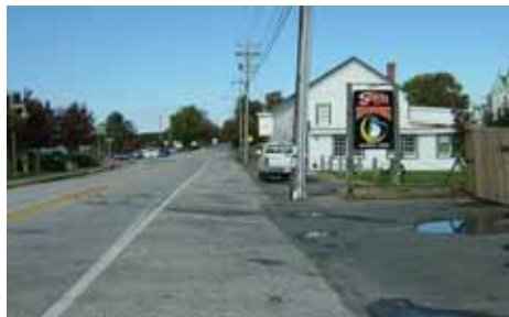
Figure 17 Existing Sidewalk Condition (non-existent)
