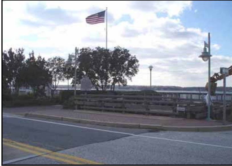
Figure 12. “TIDE BOX” BRIDGE AT THE SOLOMONS ENTRYWAY (2007)
