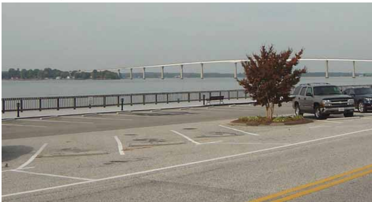
Figure 15: Existing Parking and Waterfront Condition
