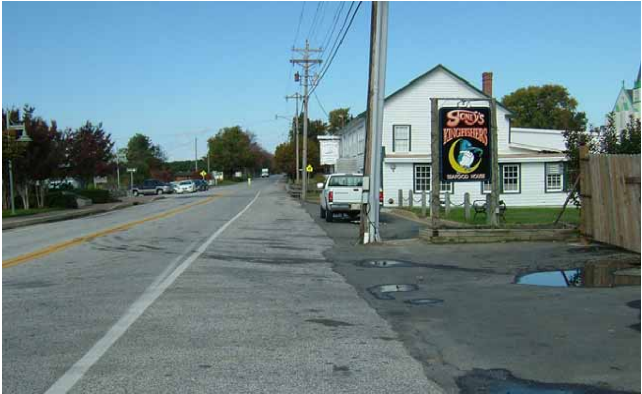
Figure 22: Existing Sidewalk Condition (non-existent)
