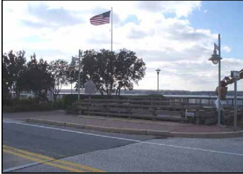
Figure 12. “TIDE BOX” BRIDGE AT THE SOLOMONS ENTRYWAY (2007)
